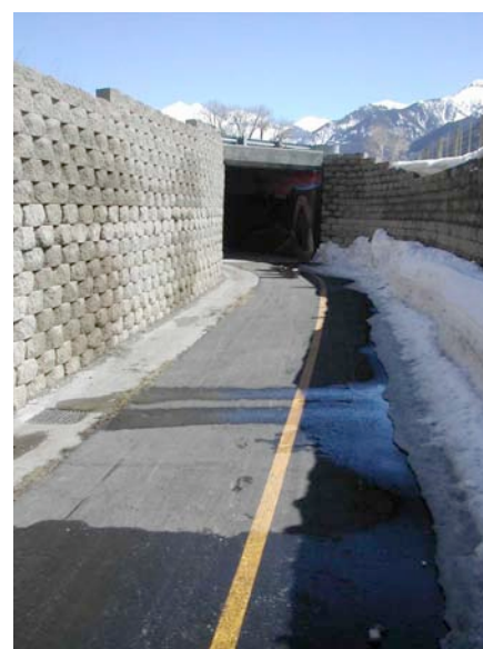
West entrance to the heated bike underpass
